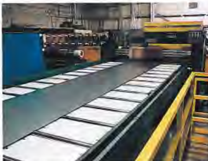
▲ Immaculate UHMW plastic runout table surface and chrome-plated rolls on low-friction bearings protect enameling and silicon electrical steels at Mapes & Sprowl Steel, Elk Grove Village, Illinois. New line slits, levels and blanks; was built by Chicago Slitter. (Photographs by the author.)
